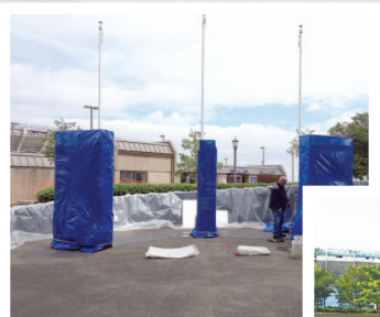
(Above) Memorial being prepared for expansion.
